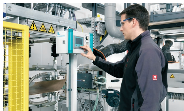
Operator panels for the most important functions are located directly at the line.
