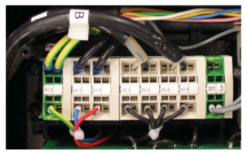
Figure 3-2. HDLC Cable Connections to Last FB ISCM Base/Redundancy Unit
